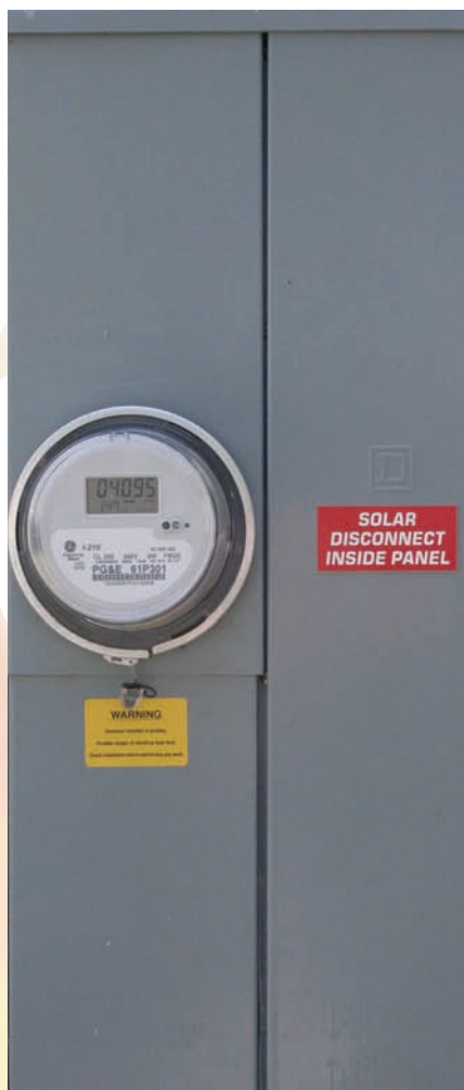
Bright, clearly labeled disconnects are important to firefighters on the scene.
