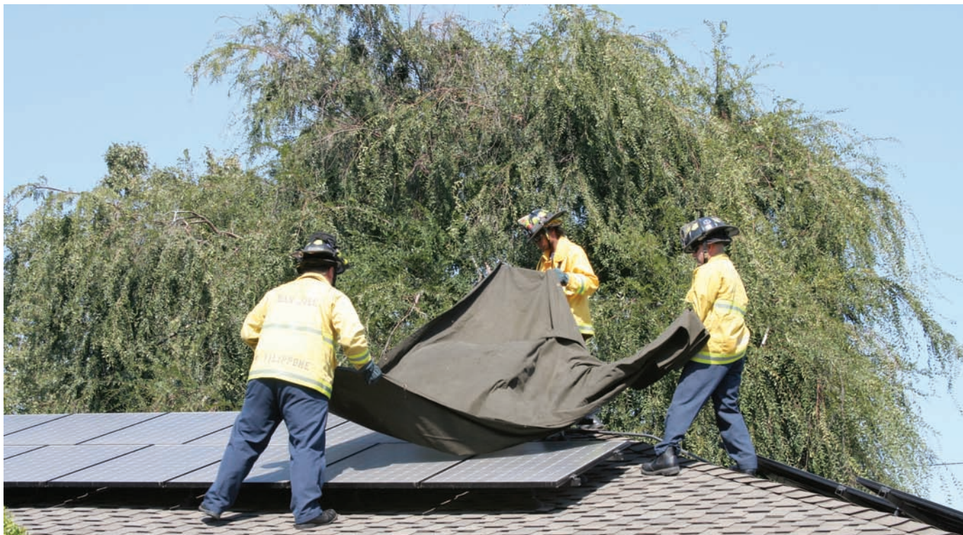
Firefighters cover a PV array with opaque tarps to cut off array power production.
