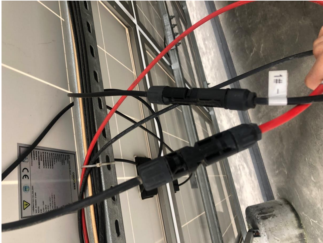
Solar Panel series connection
